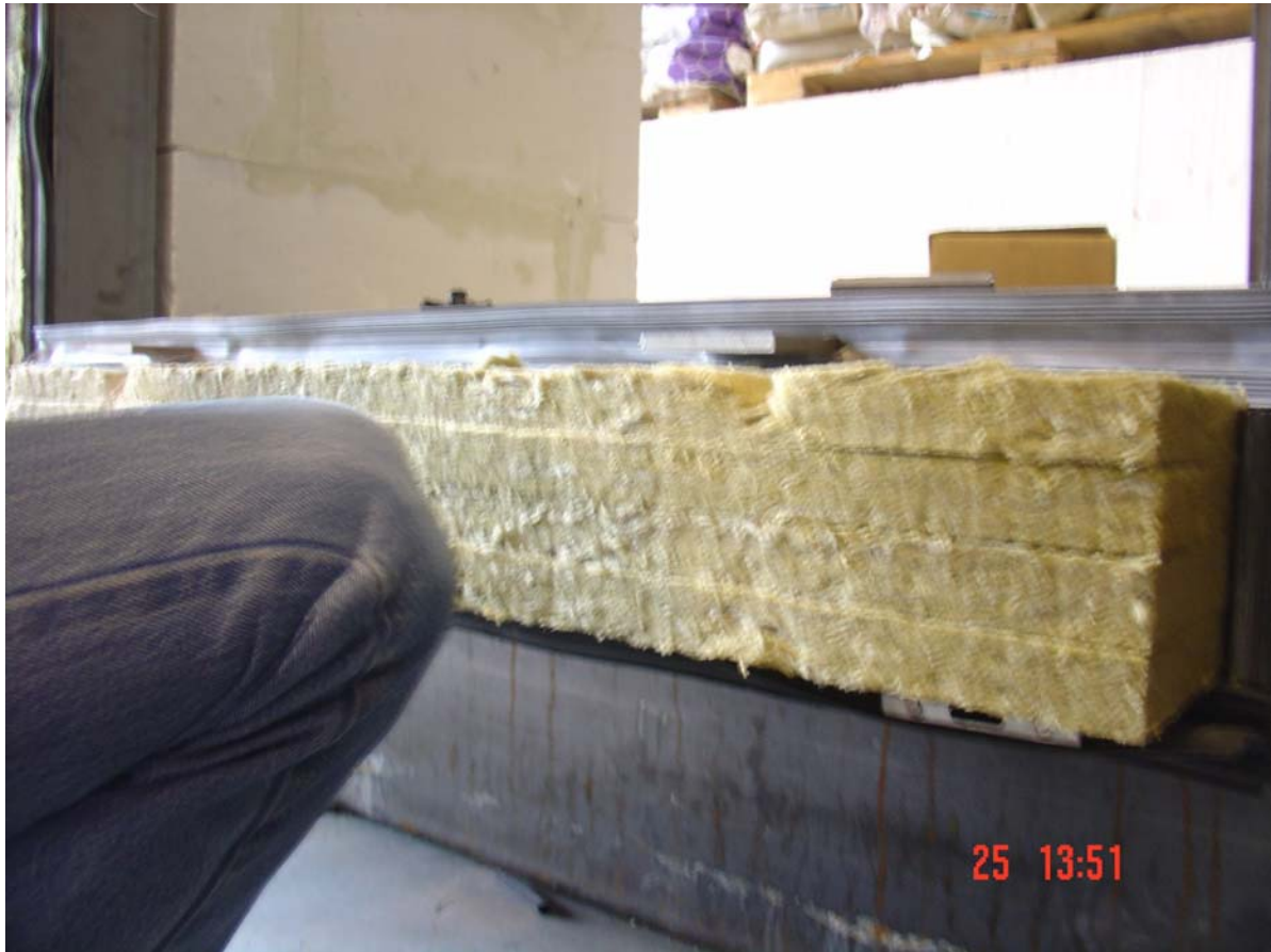
Insulation of blind facade panel
