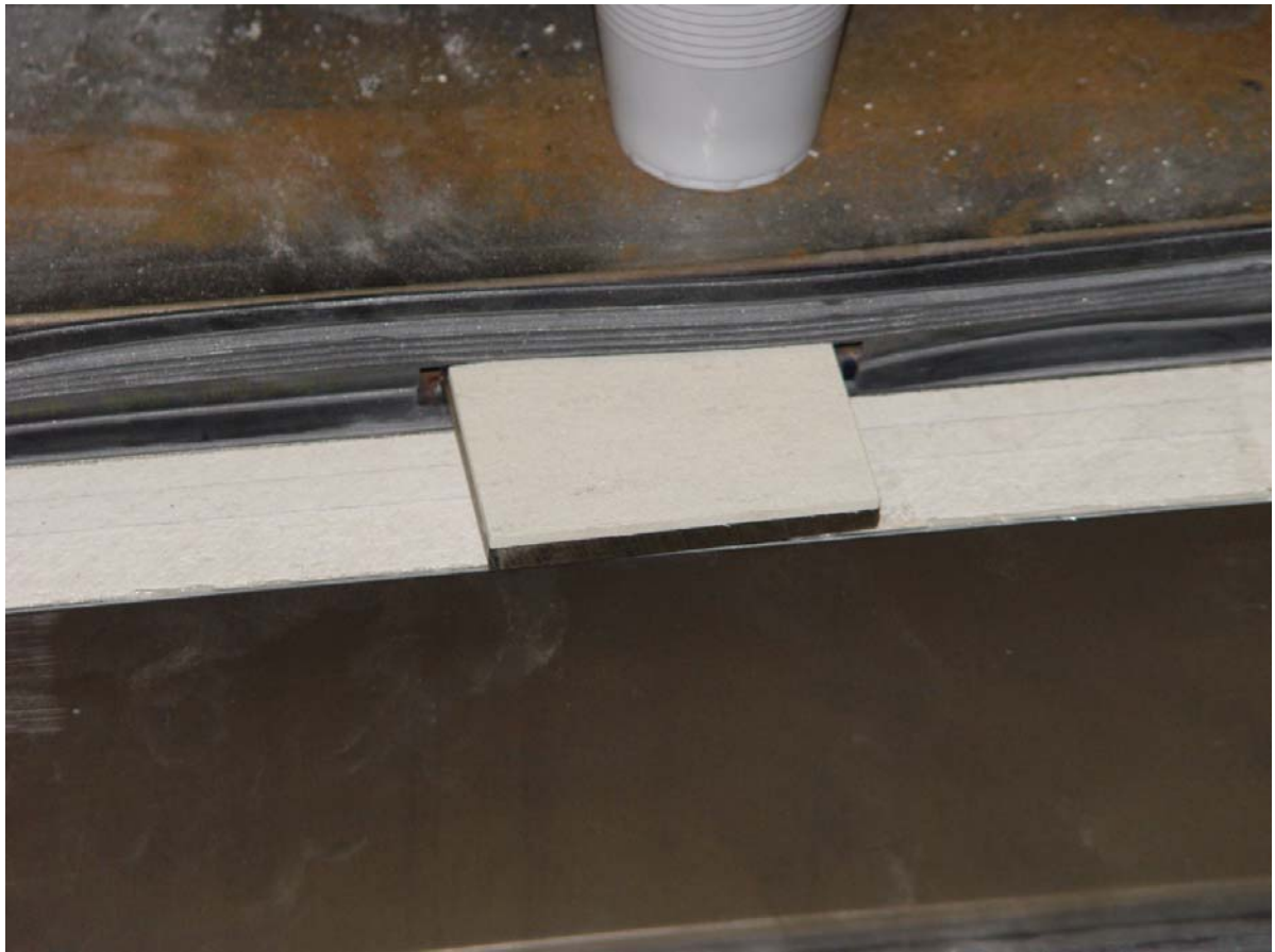
Detail of positioning strip for glazed panes
